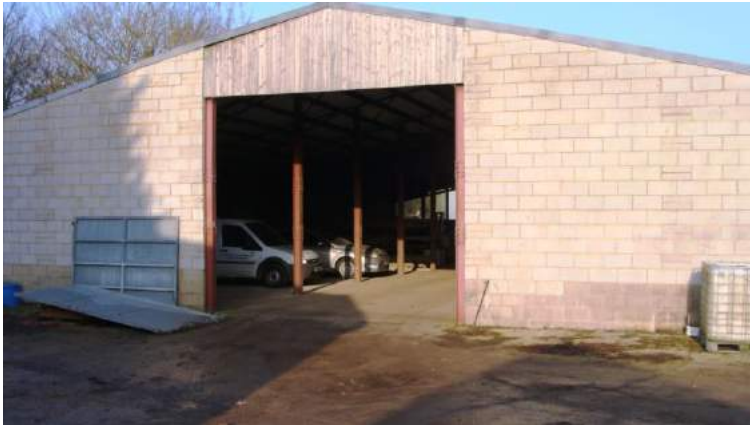
Pictures 34-35. Mid and later 20th century utilitarian buildings associated with Aspenden Hall proposed to be removed from the conservation area.
