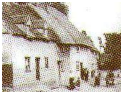
Picture 3. Cottages that were demolished to accommodate Nos. 1-8 Jubilee Cottages. What a tragedy. Source of information and reproduced courtesy of Aspenden Parish Council and their publication Aspenden at the Millennium .
