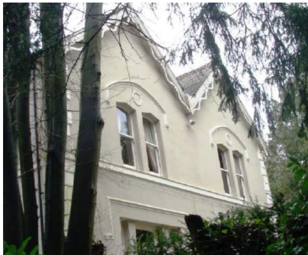
Picture 14. Good quality window surround, quoin and barge board detailing worthy of retention and protection.
