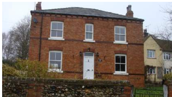
Picture 13. York House - a simply but effectively designed front elevation to this 19th century property.
