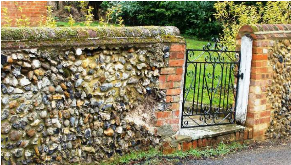
Pictures 17 and 18. Sympathetic wall rebuild and lower picture repair works required.
